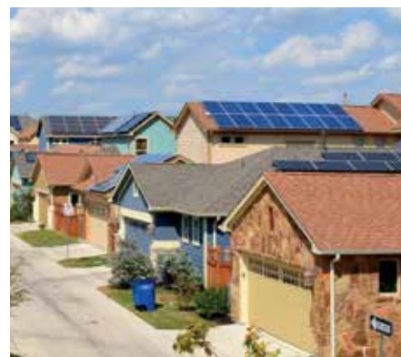
A modernized grid will promote homegrown power, as in this Austin, TX, neighborhood.
